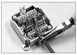
4. Using pliers, tighten the cable clamp to secure the cable to the Box.
