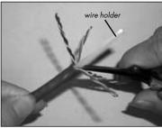
Carefully strip away approximately 30 mm of the cable jacket(s) (above left) to be connected to the Box, separating the wires into four pairs.
